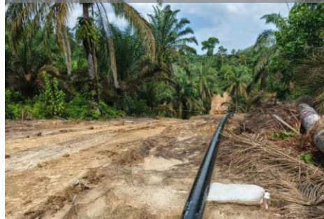
Pipe along ROW awaiting trenching May 2026
